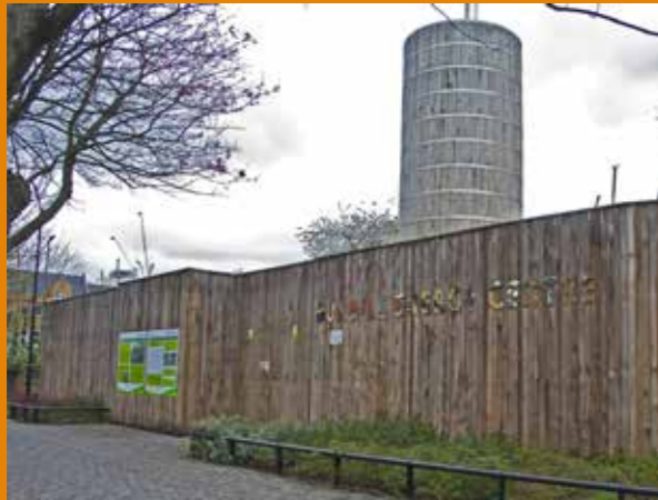
Bunhill CHP plant in Islington, London. The tower is a large heat storage unit that reduces the need to provide heat from the district heating system's backup gas boilers.
