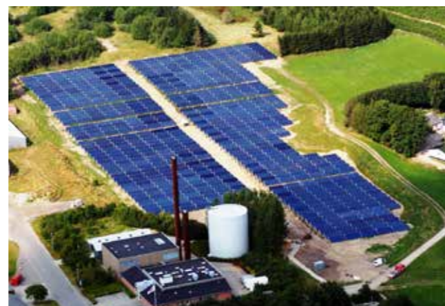
A large solar thermal plant with heat storage connects to a district heating network in Brødstrup, Denmark.
