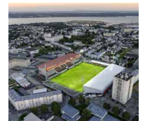
Oslo, Norway (top). Stade Francis le Blé in Brest (bottom). Connecting stadiums, leisure centres, hospitals and other anchor loads diversifies the load, making the district energy system more efficient.
