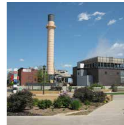
Renewable CHP plants, such as this wood-fired plant in St. Paul, USA, could provide the primary energy efficiency improvements and renewable heat that could count towards an improved efficiency label for a building.
