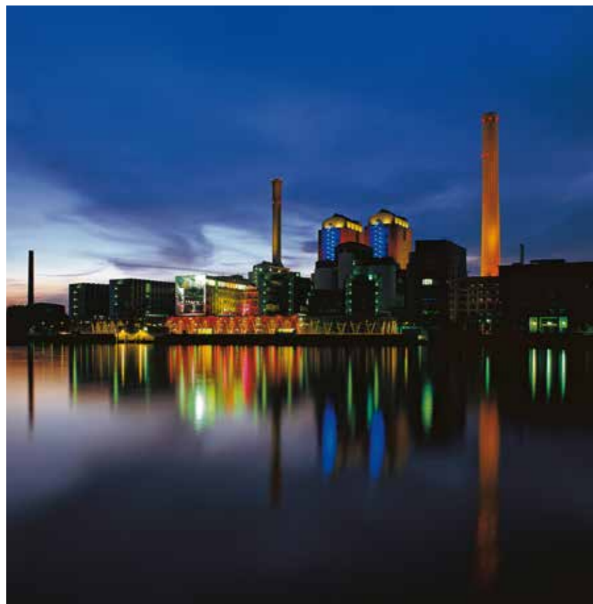
Heizkraftwerk West CHP plant in Frankfurt, Germany.
