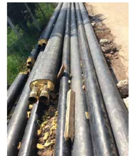
New city development in China (top). Pre-insulated district heat pipe in Botosani, Romania (bottom).
