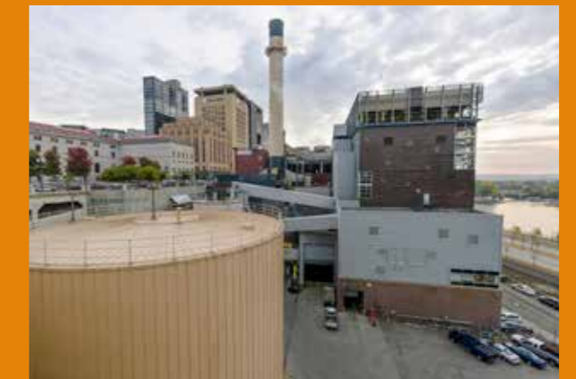
Wood chip CHP plant in St. Paul, USA.
