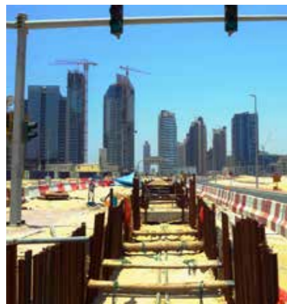
Laying district cooling pipes in Dubai, UAE.
