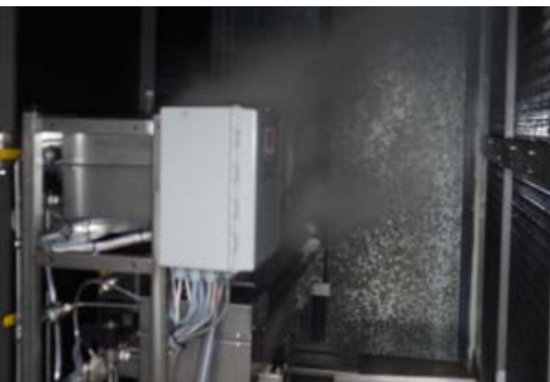
Photo: New high-efficiency ultrasonic humidifier in operation
