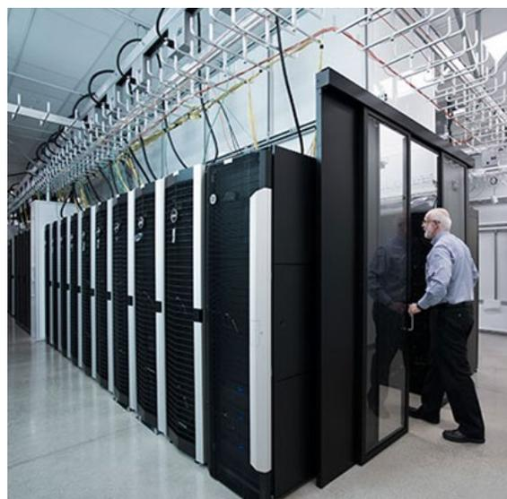
*Above- By separating hot and cold aisles and deploying outside air and chilled water for cooling, Stanford's Research Computing Facility is one of the most energy efficient locations to house servers supporting campus research.*
