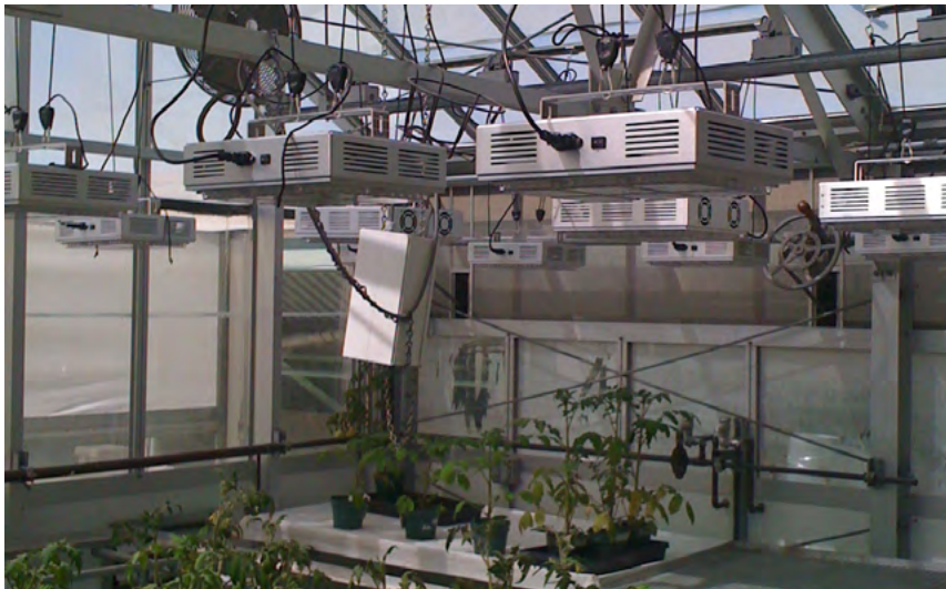
Stanford's Biology Department used ERP funds to convert greenhouse light fixtures to LEDs, saving 248,000 kwh/year.
