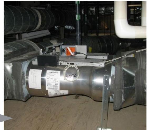
*A new Phoenix valve was installed in the interstitial space above the lab*
