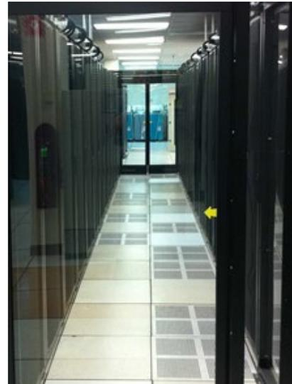
Above- A contained hot aisle of the high-density computing room prevents hot air from mixing with cool air, reducing the energy needed to air condition the room. This efficiency results in a PUE of 1.27.
