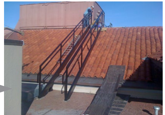
Air handler fans were reprogrammed to operate at lower speeds
