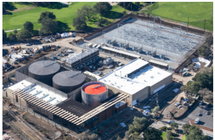
Aerial view of the new Central Energy Facility
